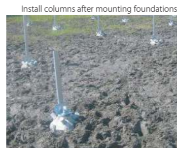
Install columns after mounting foundations
