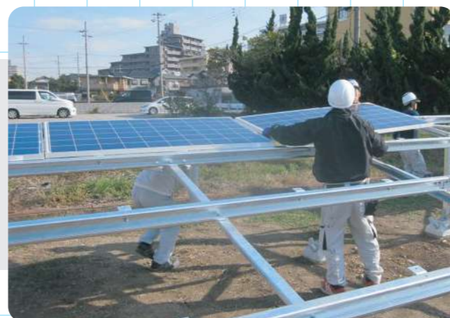
08 太陽能板安裝 Fixing Solar Panels
