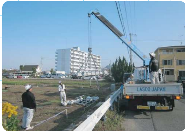
01 搬入建材 Carrying in Materials
