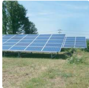
距離地面較近的施工案例 Height near to the ground level
