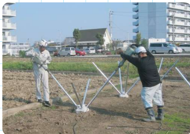
04 釘入鋼管 Driving Steel Pipes
