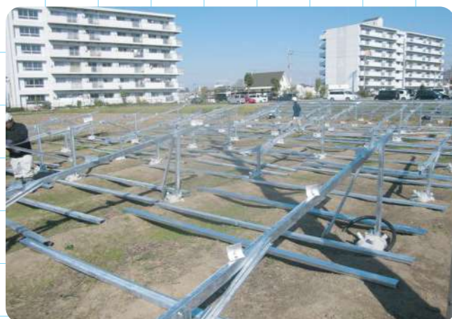
07 支架組裝 Assembling Mountings
