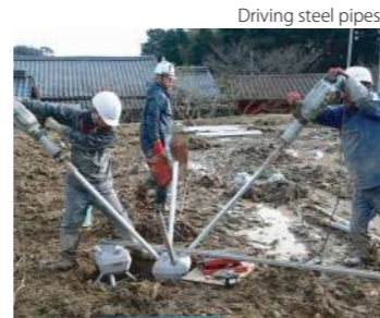
Driving steel pipes
